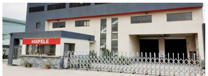
Häfele Production Plant Binh Duong, Vietnam
