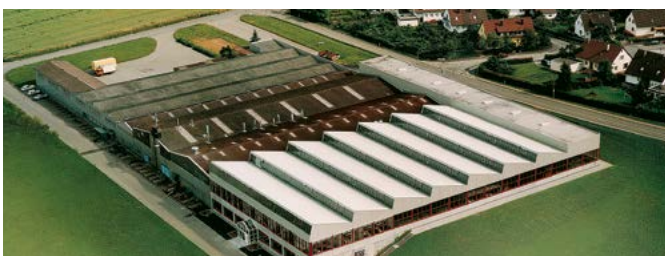
Häfele Production Plant Jettingen, Germany
