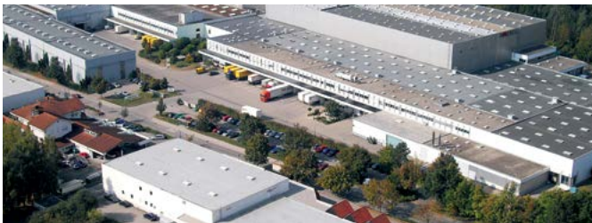
Häfele Distribution Centre Nagold, Germany
