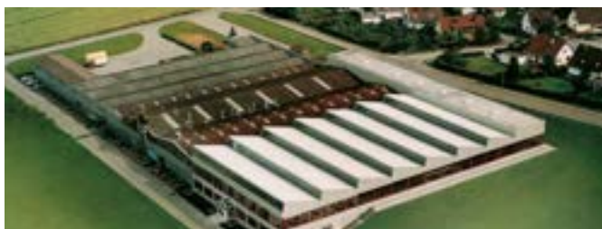
Häfele Production Plant Jettingen, Germany
